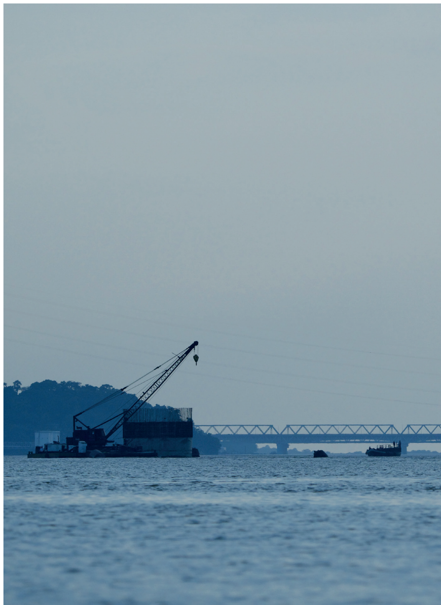
■ Bridge construction over the Brahmaputra River © Sumit Vij
