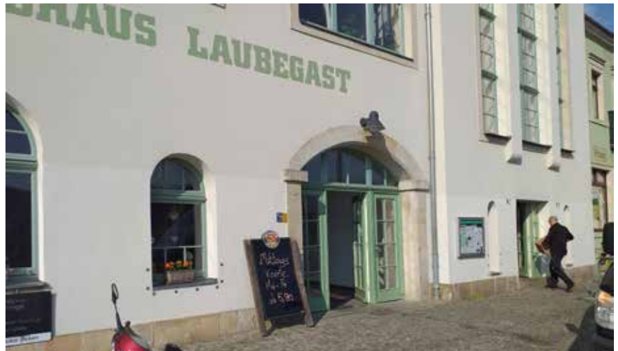
■ Bolts on the facade prepare houses for mobile barriers in case of rising water levels. Dresden, 2019. © Thomas Hartmann.
