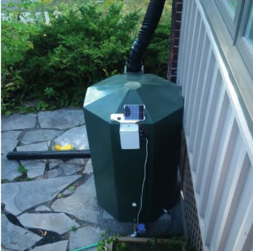
Figure 8. Stormwater Smartgrid cistern
