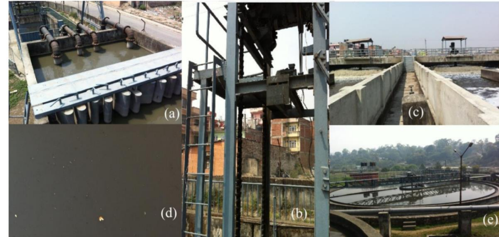
FIGURE 17. Different units of Guheshwori WWTP; (a) Usage of pump to pass the water through grit chamber; (b) Grab screen to remove large materials; (c) Blower aerators in action; (d) Feather like structures in settling tank; and (e) Settling tanks
