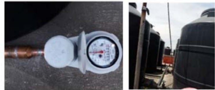
Figure 38. Micro meters installed at the low income housing of “Los Rojos” in Mexico City. Source: Josué Hidalgo, 2017
