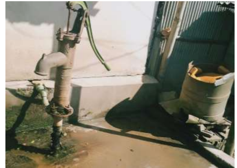
Fig: A Tube Well Source in Manohara area.
